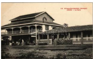
22432. ** Louga, Luga; La Gare / railway statio T1 3000
