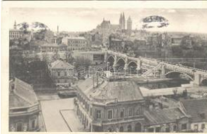
22493. ☒ 1931 Kolín, general view, bridge, rest T2 1000
