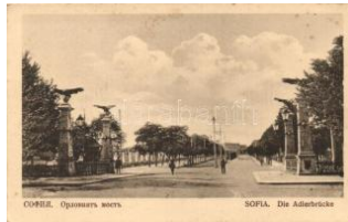
22454. Sofia, Adlerbrücke / bridge (EK) T2/3 T2/3 1400
