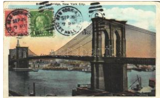
22170. ☒ 1927 New York, Brooklyn Bridge. TCV T3 1600
