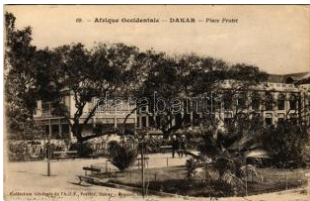
23089. ** Dakar, Place P rotet / street view T1 T1 3000
