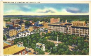
21963. ** Jacksonville (Florida), Hemmingway Park T2/3 1000
