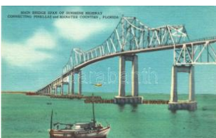
21947. ** Florida, main bridge span of Sunshine T11000
