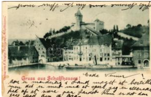
22951. 1900 Schaffhaus en, bridge, steamshi T4 1000
