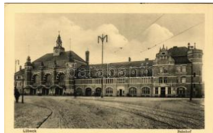
22720. ** Lübeck, Bahnhof / railway station (E T2/3 1600
