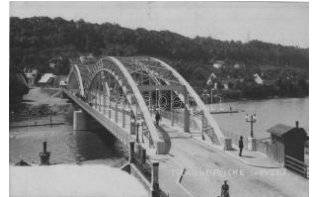
22182. ** 1901 Wels, Traunbrücke / bridge, tim T2200
