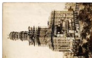
22631. * Montevideo, Construction of Palacio T2/3 1600
