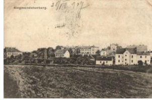
21995. 1905 Sigmundsherberg (wet damage) T3 T3 1000
