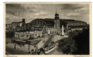
22376. ☒ 1936 Hamburg, Hauptbahnhof / railw T2/31600
