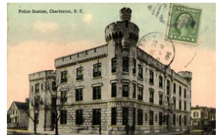
21824. * Charleston, Police Station (EB) T3 T3 2200
