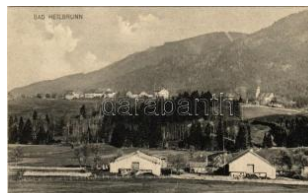
22205. 1909 Bad Heilbrunn, general view (E T2/31600
