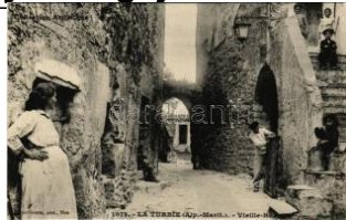
22052. La Turbie, Vieille-Rue / street view T2 T21000
