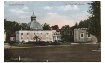
22218. ☒ Daruvar central m ud spa T2 T2 1000
