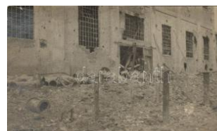
22473. * Monfalcone, WWI damaged buildings T2 2800
