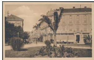
21459. * Zagreb Marovksa ulica / street, the s T1/21000
