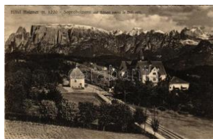
22499. ☒ 1927 Soprabolzano, Oberbozen (Sü T2/3 2000
