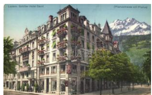
22575. * Lucerne, Luzern; Schiller Hotel Grani, T21600
