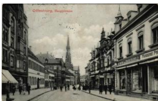
22402. 1914 Offenburg, Hauptstrasse / main T2/3 1000
