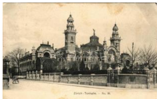
22584. ✳ 1903 Zürich, Tonhalle / concert hall (EB) T31000
