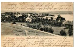
22410. 1904 Starnberg, general view, villa (p T4 1000
