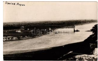
22075. * Tighina, Bender; Podul / destroyed railw T2 5000
