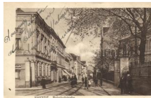
22674. Rheydt, Bahnhofstrasse / street to th T2/3 2400
