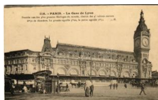
22513. Paris, La Gare de Lyon / railway station T3 1000
