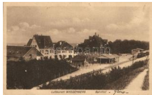
22680. * Wassenberg, Bahnhof / railway statio T2/3 2800
