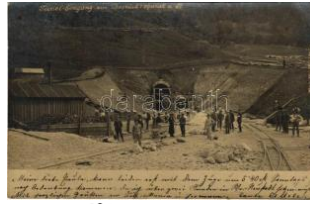
22309. 1903 Spital am Pyhrn, Tunnel-Eingang T2/38000
