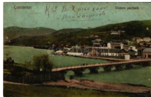
22564. * Comarnic, Komarnik; bridge (pinhole T3/43600
