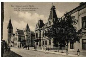
23170. ✱ Trencsénteplic, Trencianske Teplice; D T2000
