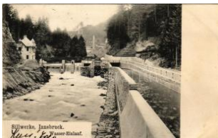
23626. 1906 Innsbruck, S illwerke, Wasser-Ein T2 1800
