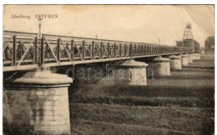
23806. * 1920 Zutphen, IJsselbrug / bridge (fa T3/4 2000
