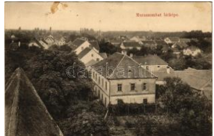
23567. 1909 Murszombat, Murska Sobota T2/3 3600
