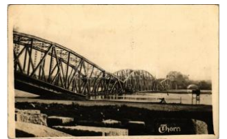
44081. 1939 Torun, Thor n; blown up bridge a T2 1600
