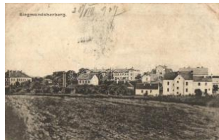
43801. Sigmundsherberg (wet damage) T3 T3 1000
