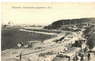
44003. ** Irkutsk, construction of railways, rail T2 2200
