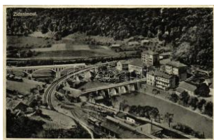
44120. ☒ 1932 Zidani Most , Steinbrück; gener T2/31600
