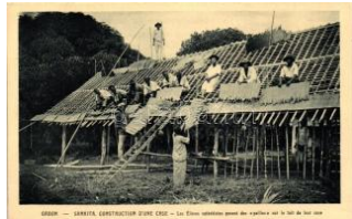
41905. ** Samkita, House construction T1 T1 2400
