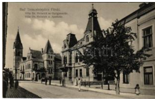
41501. Trencsénteplic, Trencianske Teplice; D T2 2000
