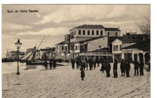
41920. ** Samos, Quai de Vathy / quay, shop T2/34000
