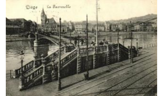
41811. ☒ Liege, Passerelle / bridge (EK) T2/3 T2/3 1600
