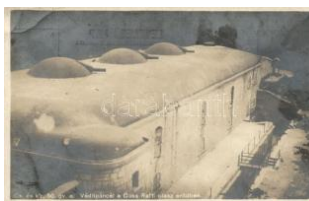
42069. ✨ Casa Ratti, fortress, security armo T2/3 3000
