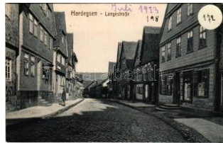
43196. * Hardegsen, Langestasse / street vie T2/31200
