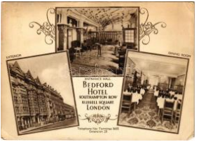
43159. 1938 London, Bedford Hotel, exterior T2/31000
