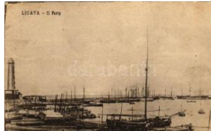
42980. ☒ 1920 Licata, Il Porto / port, lighthouse (E T3) 00
