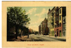
42401. Brno, Brunn; Neugasse / street vie T2/3 1200
