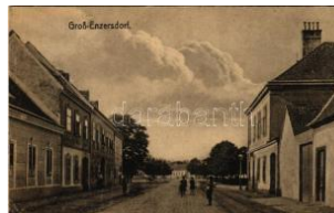
42341. 1920 Gross-Enzersdorf, Strasse / st T2/3 3000
