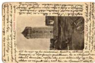
40797. ☒ 1902 Arad, víztorny / water tower (vá T46000
