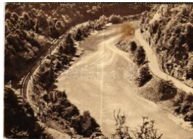
42712. * Valea Oltului, valley with railway line (T3 1600)
