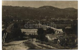
42626. Campina, bridges. Foto Olteanu, photo T2/3 2800
