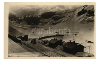
42485. Myrdal, Bergensbanen / mountain rail T2 3000
