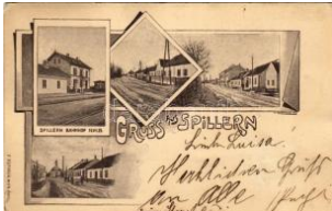
42318. * 1900 Spillern, Bahnhof / railway station T32400
