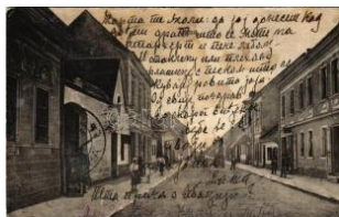
42471. * Glina, street view (wet damage) T4 T4 5000
