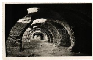
41281. ** Ada Kaleh, kata kombák / catacom T1/2 2000
