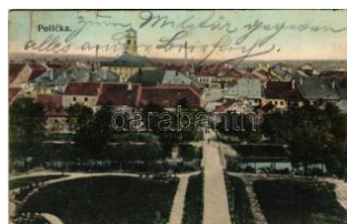
42436. 1908 Policka, general view, bridge, c T2/31200
