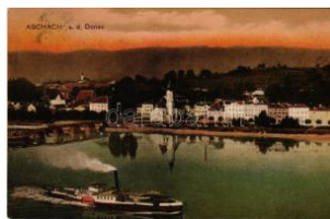
42239. ☒ Aschach an der Donau, general view T2/31600
