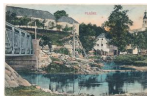
42097. * * Plaski (Lika), hí d / bridge (fl) T2/3 T2/310000
