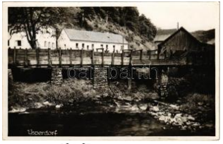
42294. ** Yspersdorf, bridge T2/3 T2/3 1200
