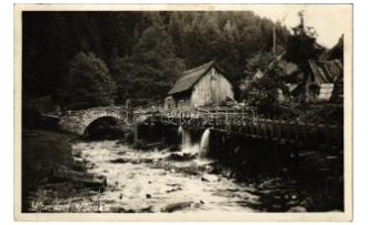
42293. 1937 Yspersdorf, bridge T2/3 T2/3 1200
