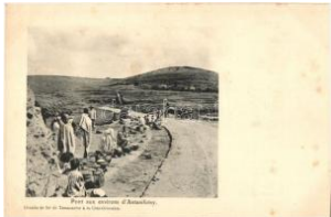
42120. ** Antanifotsy, Pont / bridge, vendors T2/32000
