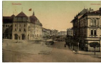
42854. ☒ Szabadka Eötvös street (wet damag T3/4 1200
