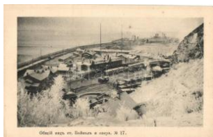
43635. * Port-Baikal, Baykal (port); station of th T22200
