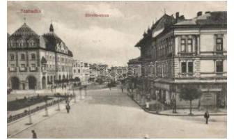
42852. ☒ Szabadka Eötvös street (wet damag T3/4 1200
