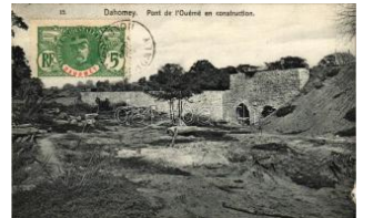
43300. * Ouémé, Pont en c onstruction / bridge c T13000
