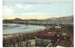
43492. ** An-hai (Anping) bridge T1/2 T1/2 2000
