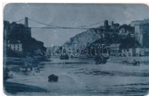
42392. ** Bristol, Clifton Suspension Bridge T2 T21400
