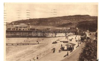
42402. ☒ Colwyn Bay, promenade and pier (EK T2/31400
