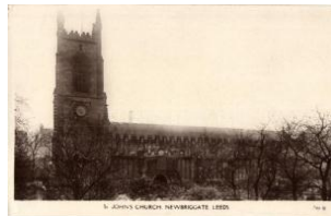
42413. ** Leeds, New Bridge, St. John's Church T2 1400
