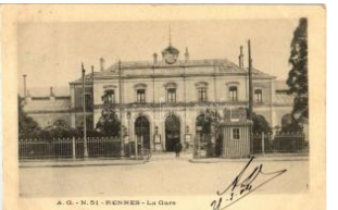
42331. ☒ Rennes, La Gare / railway station T2 T2 3000
