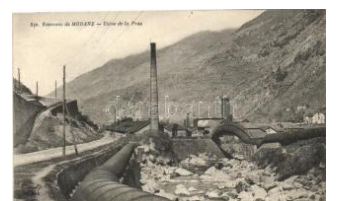
42302. ✳✳ Modane, Usine de la Praz / factory T 22000
