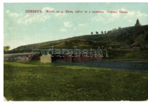
42393. * Plevn, bridge on the River Vit, whe T2/3 1000
