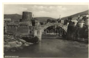
42358. Mostar, Stari most / bridge T1/2 T1/2 1000
