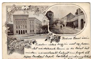
42357. 1902 Mostar, Gymnasium, Hauptstrass T3 4000
