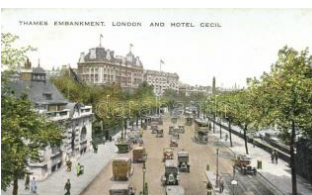
42516. ☒ London, Thames Embankment, Hotel Cecil T2/3 1000
