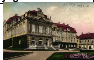
42427. ✱ Lysá nad Labem (wet damage) T4 T4 1000
