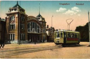
42241. * 1913 Klagenfurt, Bahnhof / railway stati T3 2000
