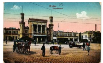
42101. 1920 Wrocław, Breslau; Hauptbahn T2/33000
