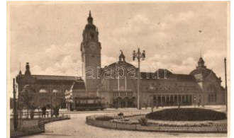
42233. Wiesbaden, Hauptbahnhof, railway T2/3 1200
