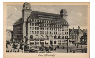
42121. Essen, Hotel Handelsloshof, restaurant T2/31400
