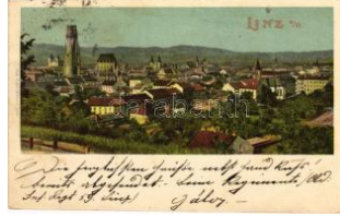
42000. ☒ 1901 Linz a. Donau (wet damage) T2/3/1800
