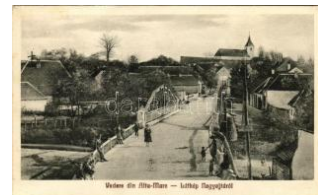
41870. 1941 Nagyajta, A ita Mare; hid / bridge T26000
