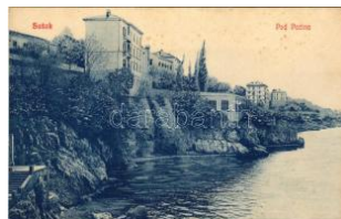
42813. ** Fiume, Rijeka; Susak, Pod Pecina ( T2/31800
