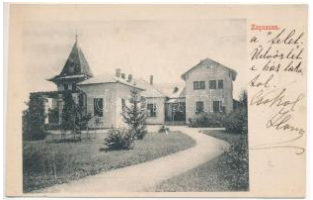
42275. 1909 Zaguzsén, Zagujeni (Temes) T2/3 22000
