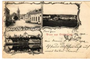
42957. 1900 Ottensschlag, street view, castle T2/32000
