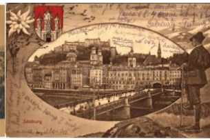
42965. 1915 Salzburg, bridge, tram, castle. T2/3 1600
