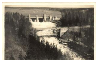
42344. ** Imatra, river da m, bridge T2 T2 1400
