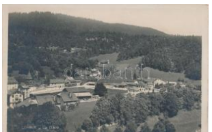
42498. Saint-Cergue, Gare / railway station T2 1200
