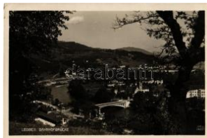
42168. ☒ Leoben, Bahnhof brücke / railway sta T1/21400
