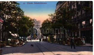
42526. ** Zürich, Bahnhofstrasse / railway station T1/2 1400
