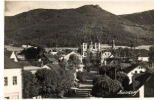
42292. ☒ Hajnice, Haindorf; street, church, au T2/3 1400
