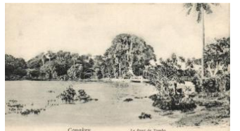
42498. ** Conakry, Le Pont de Tombo / bridge T1/2 1000
