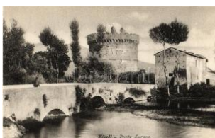
42795. ** Tivoli, Ponte Lucano / bridge, tower T2 1400
