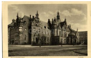
42644. ** Leipzig, Buchhandlerhaus / building T1 2000
