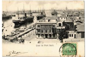
42400. 1906 Port Said, Quai / dock, ships. T T2/3 1600
