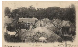
42905. * 1902 Dakar, Fortier / village, huts (R T2/31000
