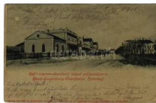
40837. * 1915 Sopron, Győr-Sopron-Ebenfurti V T37500
