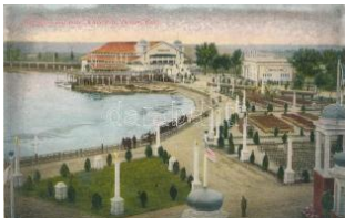
42280. ** Denver, Colorado; Ball Room and Library T21200
