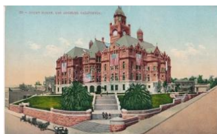
42298. ** Los Angeles, California; Court House T2 1200
