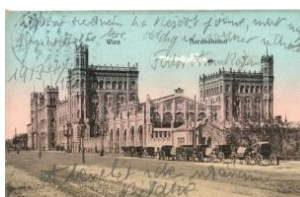
42544. Vienna, Wien; Nordbahnhof / railway station T41000
