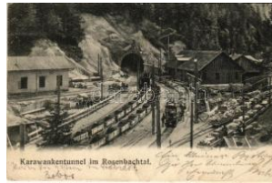
42502. Rosenbachtal, Karawankentunnel / K T2/3 3000
