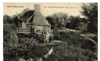
42843. Dol-de-Bretagne, Moulin / mill T2 T2 1200
