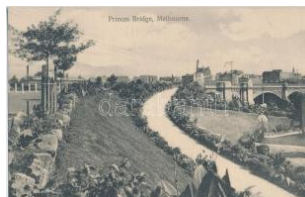
42409. ✨ ✨ Melbourne, Princess Bridge T1 T1 1200
