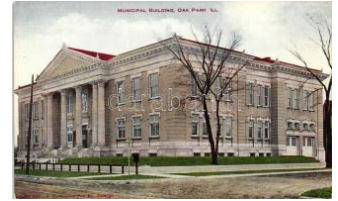
42343. ** Oak Park, Municipal building T2 T2 1000
