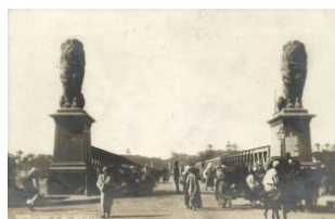
42773. ** Cairo, Kasr-El-Nil bridge T2 T2 1400
