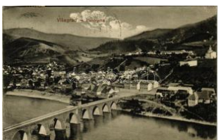
43093. 1915 Visegrad, g eneral view, bridge T2/33000
