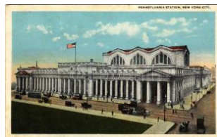
43966. New York, Pennsylvania railway sta T2/32000
