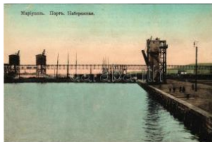
44186. ✳✳ Mariupol, port and bankment, indus T1/2 2000
