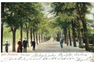
41998. ☐ Bad Nauheim, Park Allee T2 T2 1200
