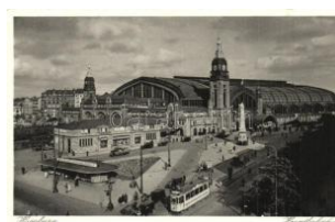
42035. ** Hamburg, Haup tbahnhof / railway sta T2 1000
