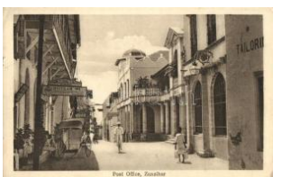
42579. Zanzibar, Post Office, street, shops T2/3 1800
