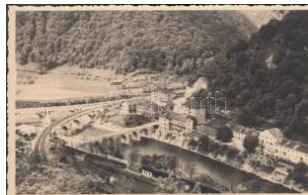
42572. Zidani Most, bridge T1/2 T1/2 1400
