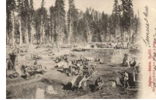
42425. ☒ Taiga, Constructi on workers T2 T2 4000
