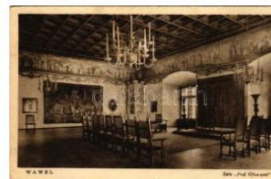
42386. Kraków, Krakau; Wawel, Sala Pod T2/3 3000
