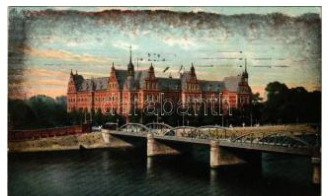
42482. * 1909 Wrocław, Breslau; Lessingbrücke T2/3 3000
