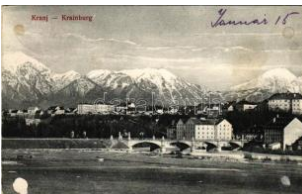
42845. ☐ Kranj, Krainburg; general view, brid T2/3 2600
