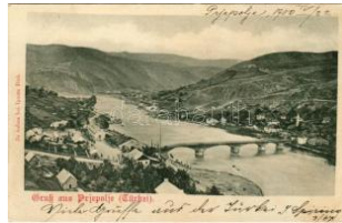
42655. * 1900 Prijepolje, general view, bridge T2/31600
