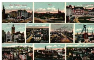
42387. Ostrava, Morav ská Ostrava, Máhrisc T2/300
