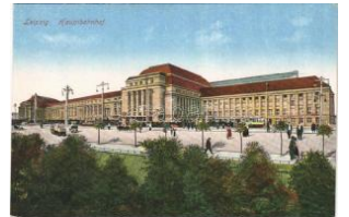
43478. ** Leipzig, Hauptbahnhof / railway station T1 1600
