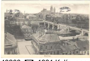
43203. 1931 Kolín, general view, bridge, rest T2 1000
