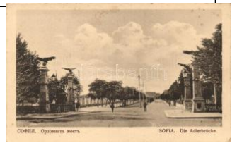
43154. Sofia, Adlerbrücke / bridge (EK) T2/3 T2/3 1400
