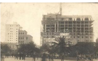
22032. 1925 Vitória, Victoria; Building construct 3000
