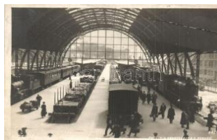
22359. Bergen, station / Bahnhof / railway st T3 2400
