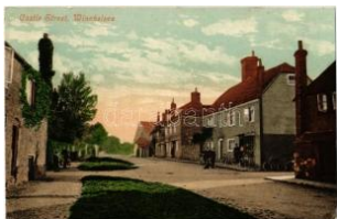
22334. 1904 Winchelsea, Castle street, shop, bicy T2 2400
