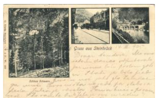
22866. 1905 Zidani Most, Steinbrück; Schlo T2/38500
